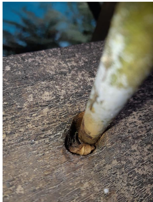
Figure 16. Typical view of sheltered corrosion of hanger rods through treated timber transoms with unknown section loss deeper in timber section.
