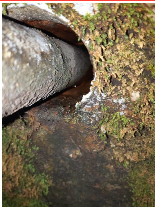
Figure 7. Example of the anchor rods in their tube fixed into the concrete mass block
