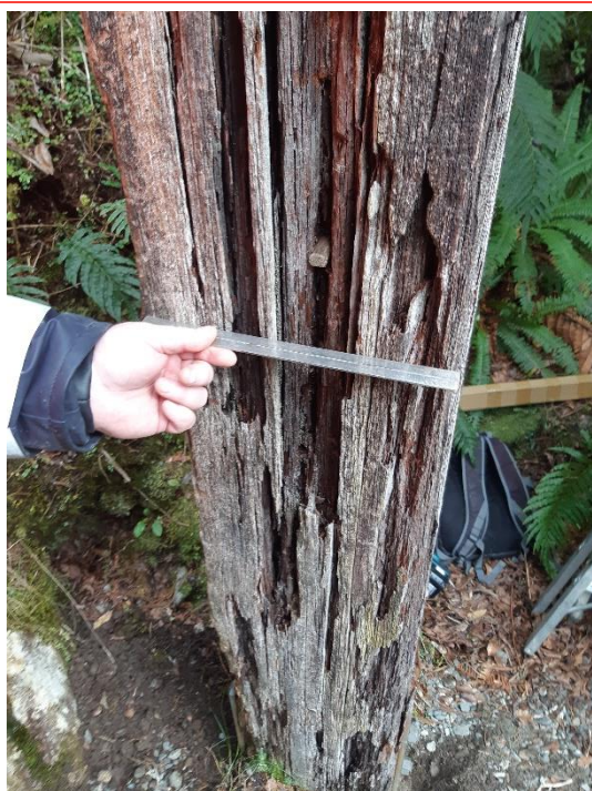
Figure 3. Upstream Abutment A tower support showing surface decay pockets up to 30mm
