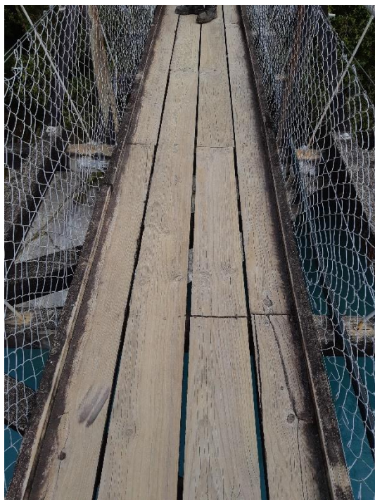
Figure 9. General view of deck condition noting polished surface and plank end cracking
