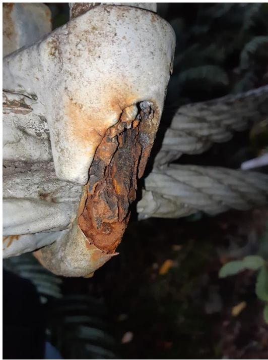
Figure 13. Older clamps exhibiting section loss and requiring replacement
