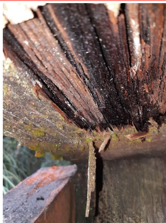
Figure 4. Upstream Abutment A tower cap soffit showing surface decay pockets up to 15mm with white spot
