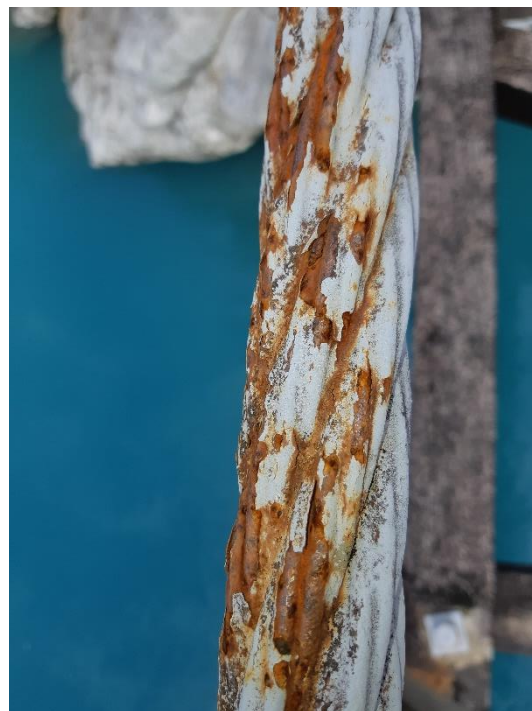
Figure 10. Main cable condition noting isolated pitting in strands and previous repair coating delaminating and cracking
