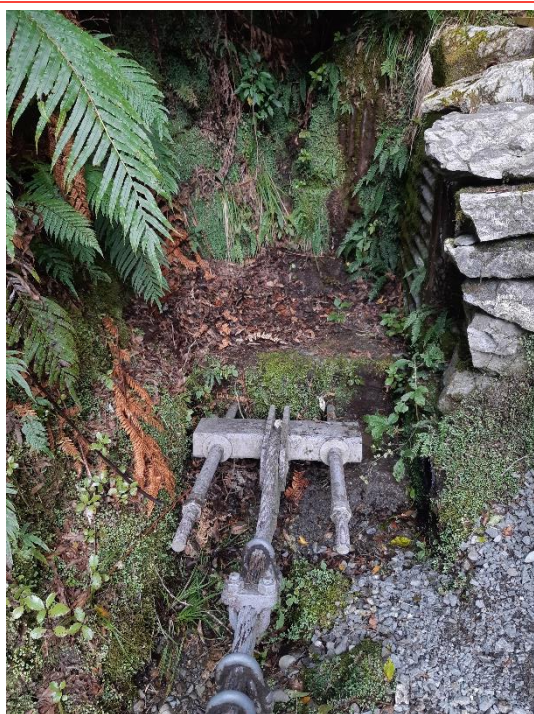
Figure 5. General view of tower anchor assembly Abutment A (true right) downstream
