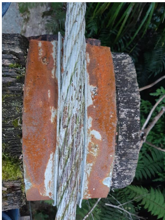
Figure 11. Typical condition of the main cable saddles at tower tops showing general corrosion and spreading of the cable due to no side support in the sheave
