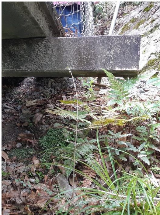
Figure 17. Slack requiring adjustment in hanger rod
