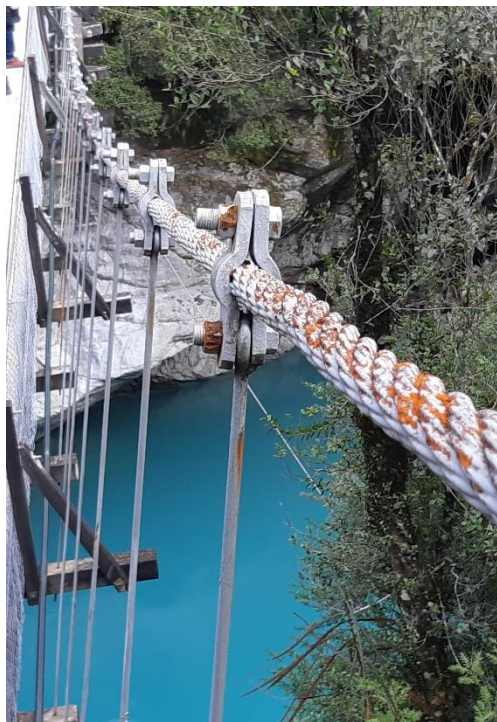
Figure 13. Older clamps exhibiting section loss and requiring replacement
