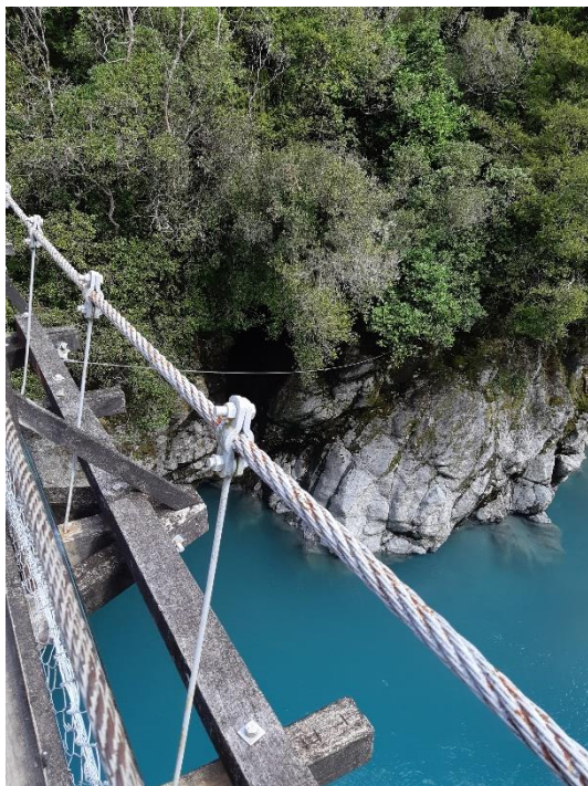
Figure 17. Slack requiring adjustment in hanger rod
