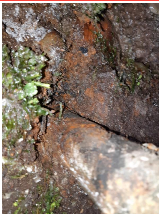
Figure 8. Example of anchor rod where corrosion is visible outside the cast in tube
