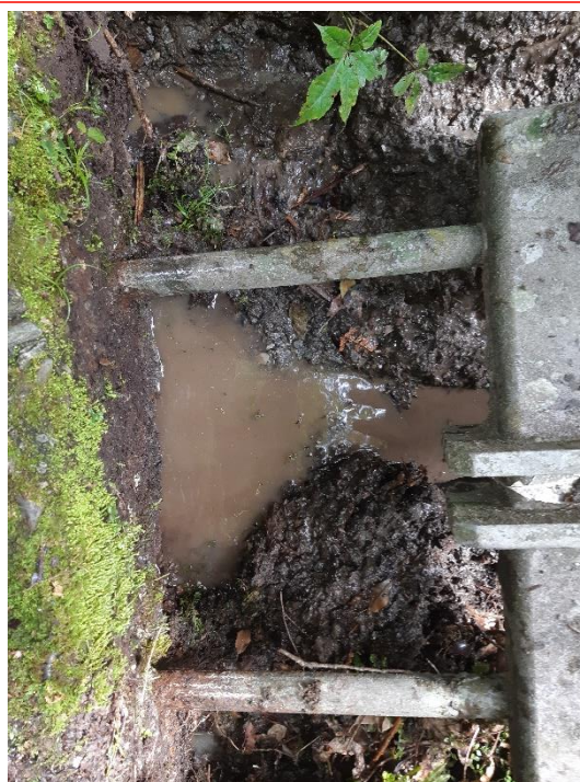
Figure 6. Water flowing out from anchor block to assumed bed rock level
