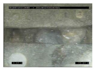
42\_20120524161016us\_SV\_.jpg, 00:21:13, 76.25m (10.96m) The soil or trench material outside the pipe is visible through a defect from 7 o'clock to 3 o'clock / Gravel visible in open joint
