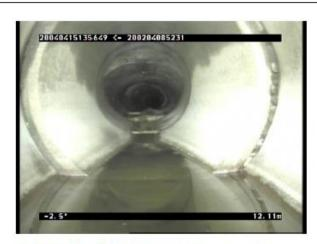
1020040415135626dsJDVS12.11.jpg, 00:04:30, 12.11m (4.31m) Joint vertical displaced, less than 10% of pipe diameter
