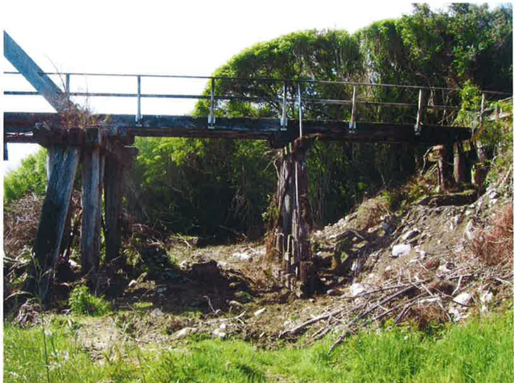
Figure 4-2 : Typical End Span (Spans 8 and 9 – Southern End)
