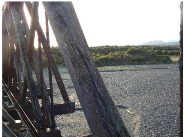
Typical Timber Splitting – King Strut Shown.
