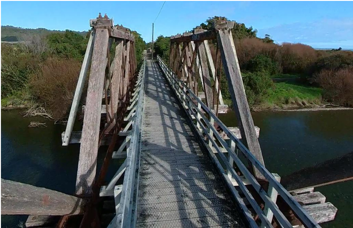
Figure 3: Deck Approach of Totara Bridge.
