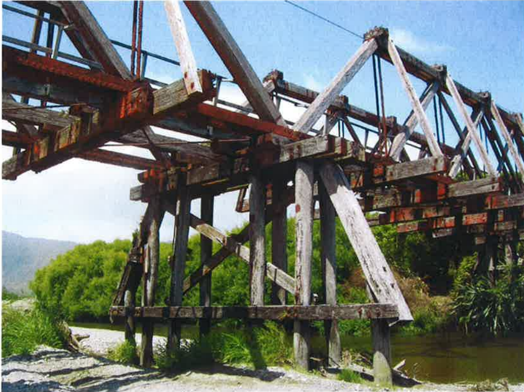
Figure 4-3 : Typical River Pier (Pier No. 7)
