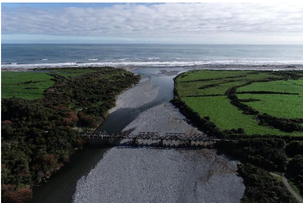
Observation – Flow Favours True Left of River as this is the Outside of the Curved Alignment. Significant Gravel Deposition.
