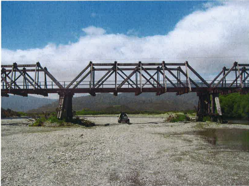
Figure 4-1 : Typical Howe Truss Span (Span 6 – Downstream)
