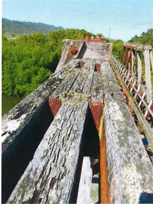
Figure 5-1 : Top Chord of Timber Trusses – Minor Weathering / Splitting Only, “Sound”
