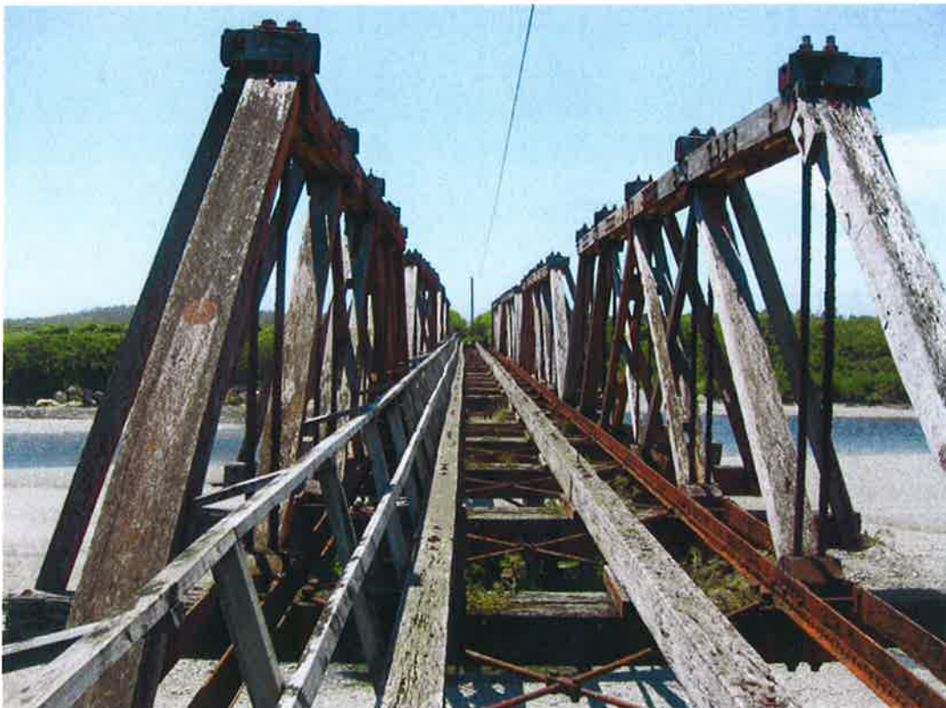
Figure 4-4 : Typical View North Along Bridge
