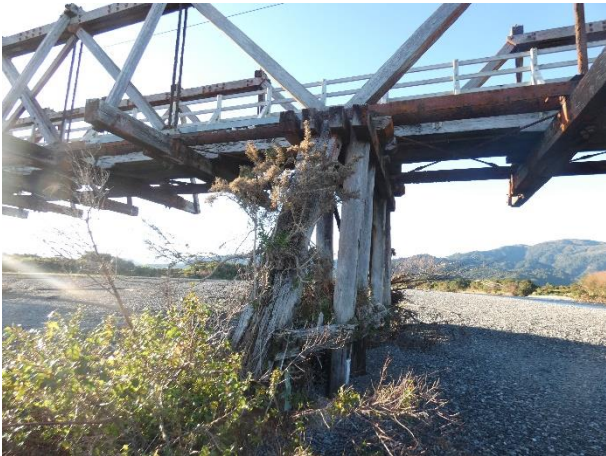
Vegetation Growth From Timber Decay Pockets
