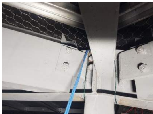
Photo 6 – Internal view of roof valley beam connections
