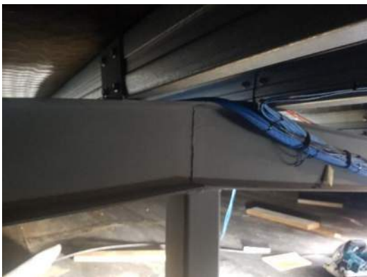
Photo 5 – Internal view of main portal rafter at roof level.
