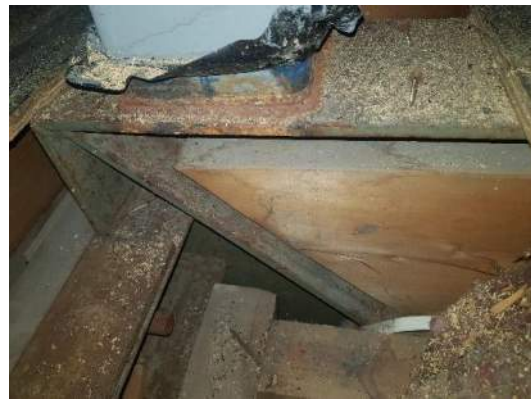
Photo 4 – internal view to portal knee connection at second floor ceiling level
