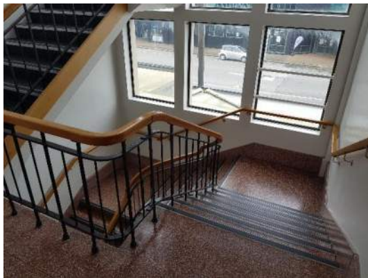
Photo 3 – Internal view (southern staircase)
