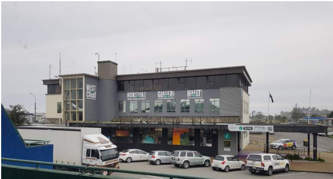
Figure 1. View of building (Southern elevation)– from weld street.
