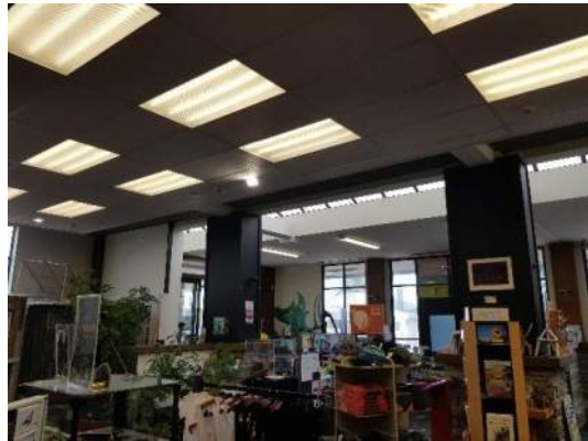
Photo 2 – Internal view to library extension to south end circa 1990
