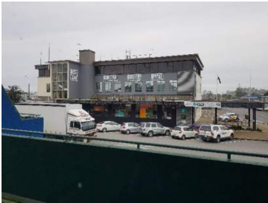
Photo 1 – Exterior view to southern elevation of building.
