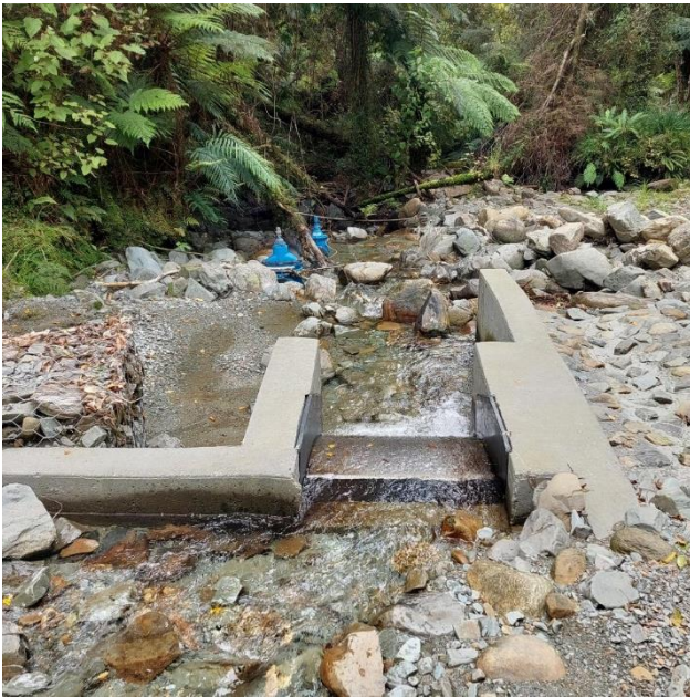
Figure 4-5: Intake Weir.
