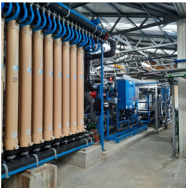
Figure 3-7: Membrane Skid.
