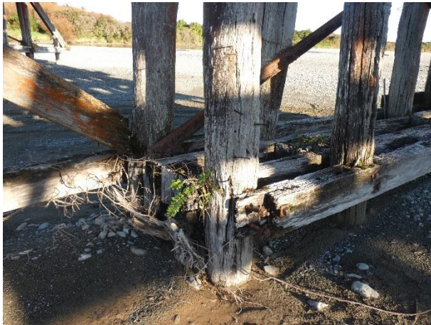
Missing Pier Waling Timbers
