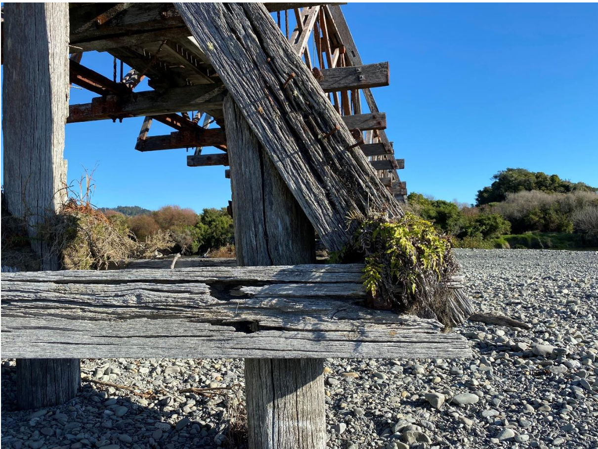
Timber loss and decay.
