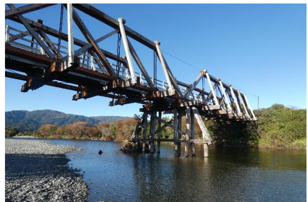
Pier G and Underside of Span G-H not inspected due to Channel Location. Main Channel is Deep. Pile Embedment Depth Unknown.
