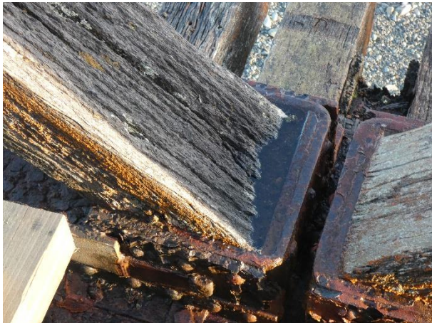
Typical Weathered Timber and Ponding Moisture.
