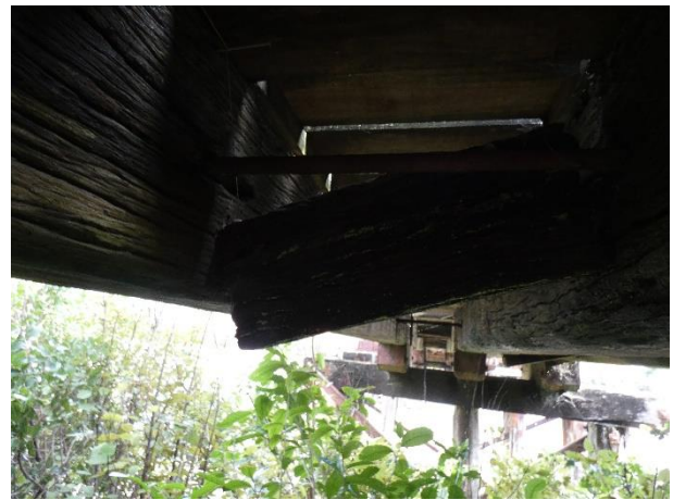
Dislodged and Missing Timber Bracing Blocks Typical.
