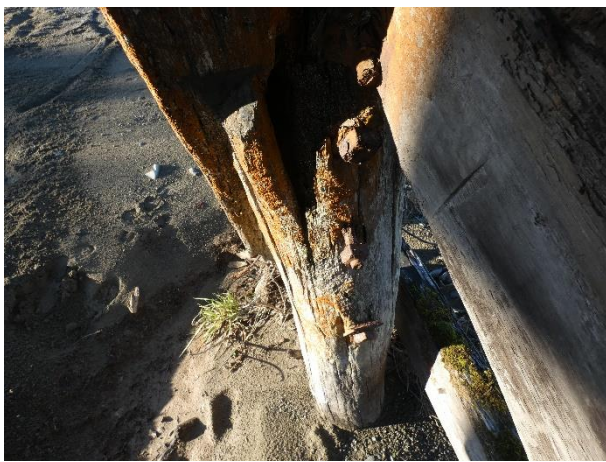
Typical Decay of Pier Piles
