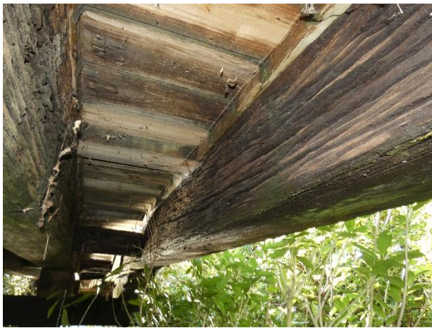
Moisture in Timber Components. Reduced Air Flow for Drying due to Vegetation.
