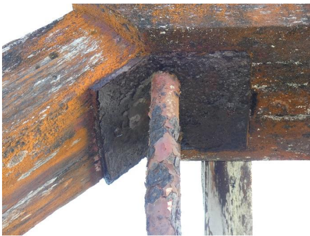
Corrosion of Truss Connection Plates.
