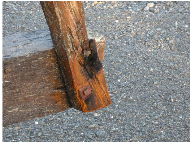
Typical Decay and Loss of Timber Section at Connections – Bottom of Wind Brace Shown.
