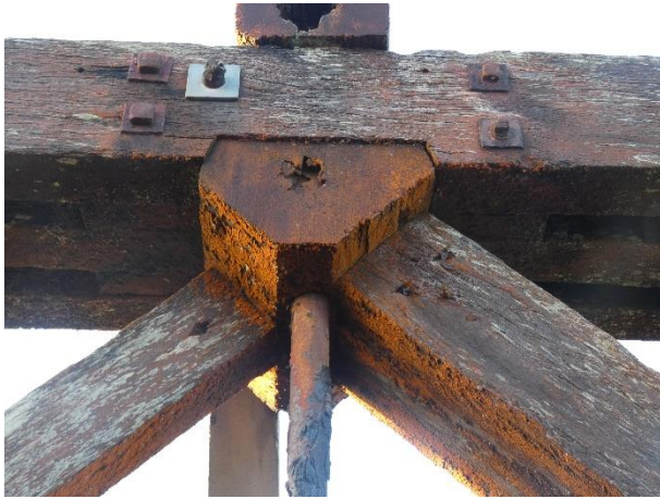
Typical Moderate Decay of 'A' Block.
