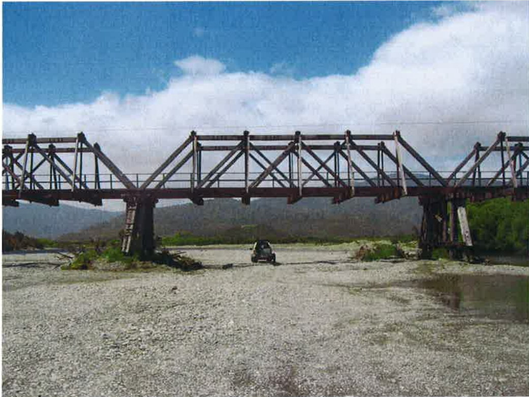
Figure 4-1 : Typical Howe Truss Span (Span 6 – Downstream)
