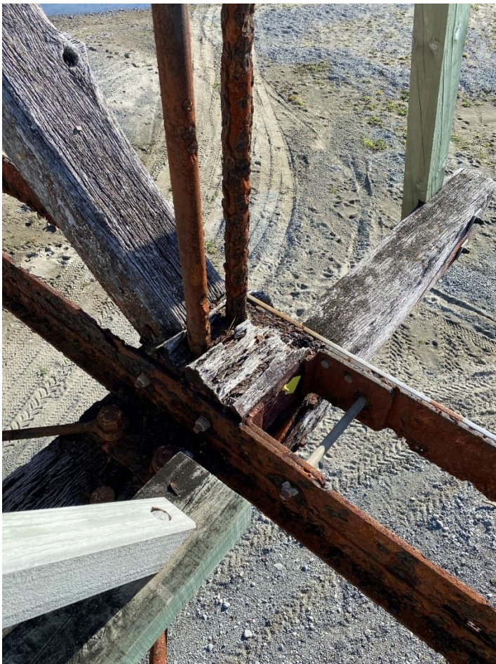
Timber thrust block with timber decay.
