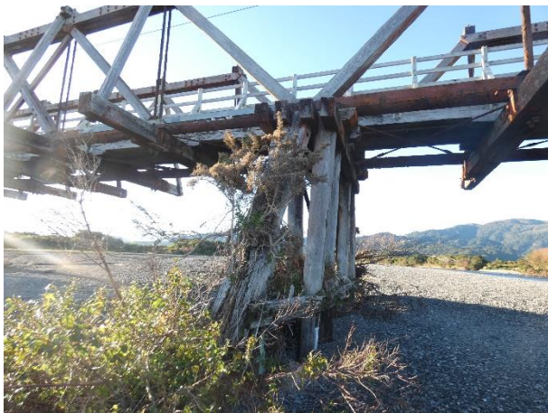
Vegetation Growth From Timber Decay Pockets
