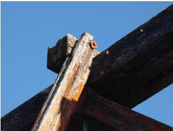
Typical Decay and Loss of Timber Section at Connections – Top of Wind Brace Shown.
