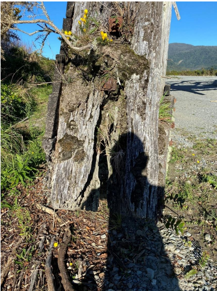
Raking pile timber split and timber decay.
