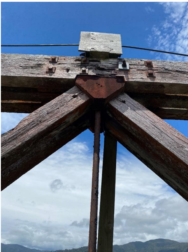
Saddle block needs replacing.
