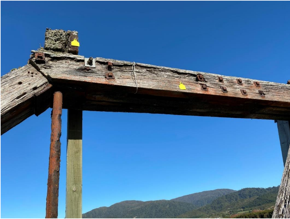
Top Cord Surface loss Saddle block split in timber and timber decay.
