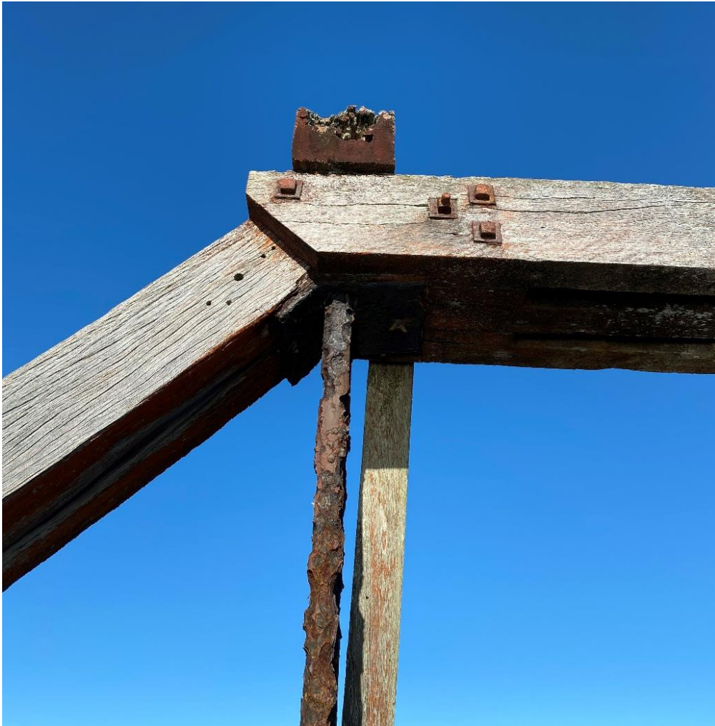
Saddle block timber decay. Tension rod corroded.
