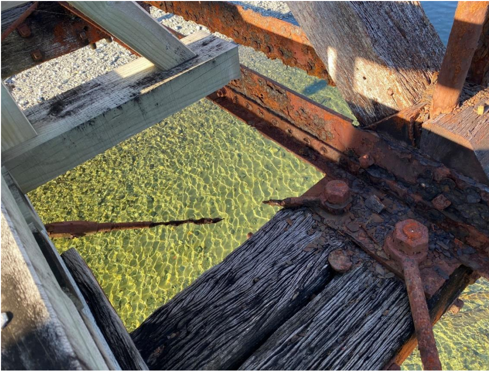
Steel cross bracing corroded. Needs replacing
