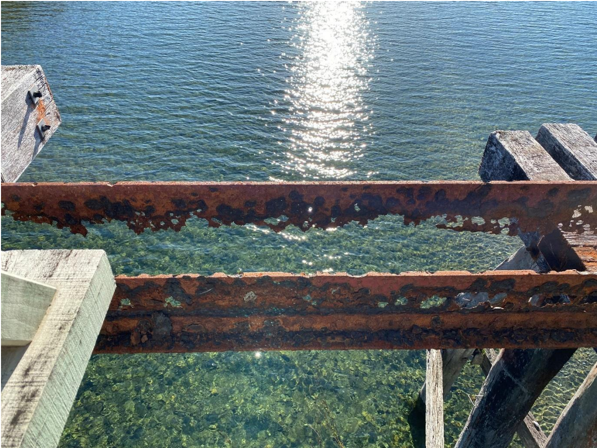
Bottom cord corroded. Needs replacing.
