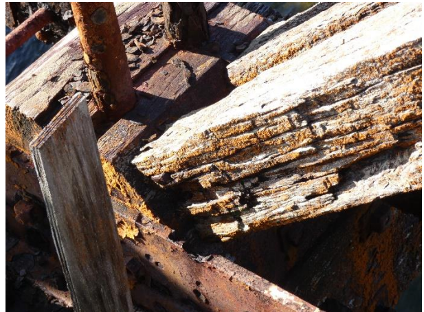
Typical Weathered Timber.
