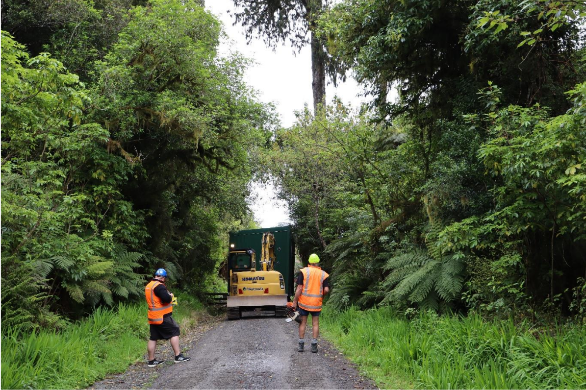
Figure: Fox Glacier Treatment Plant arrives on site (commissioned November 2023).
