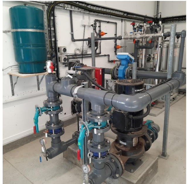
Figure 6-6: Reticulation Pumps.
