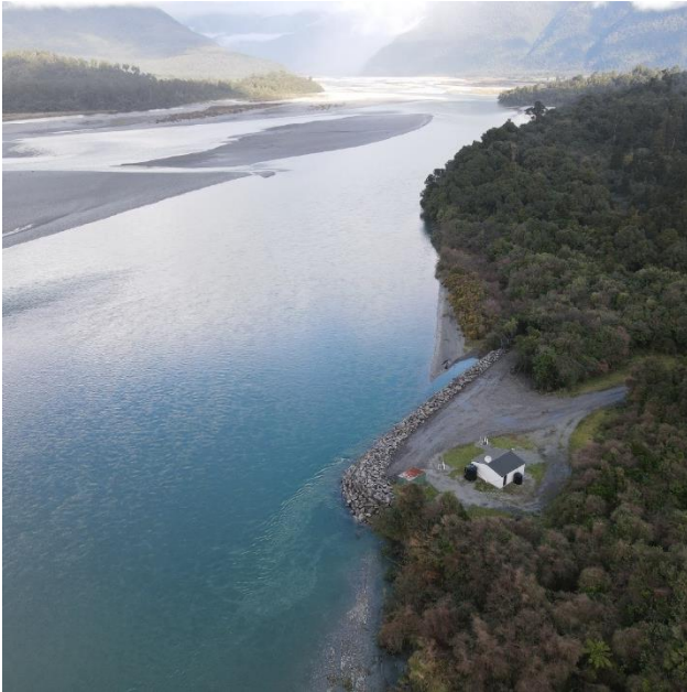
Figure 9-5: Location of Treatment Plant.
