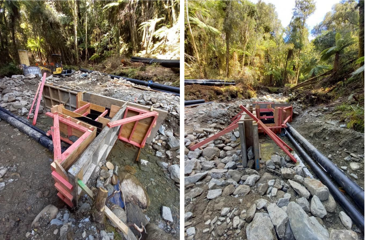
Figure: Construction of the Ross Water Supply Intake (March 2022).
