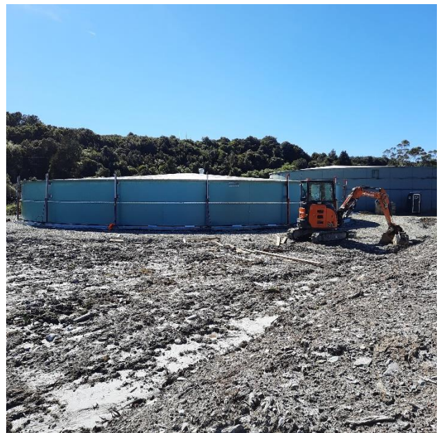
Figure 3-8: Reservoir at Treatment Plant.
